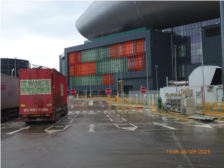
Staff parking area looking towards office block
